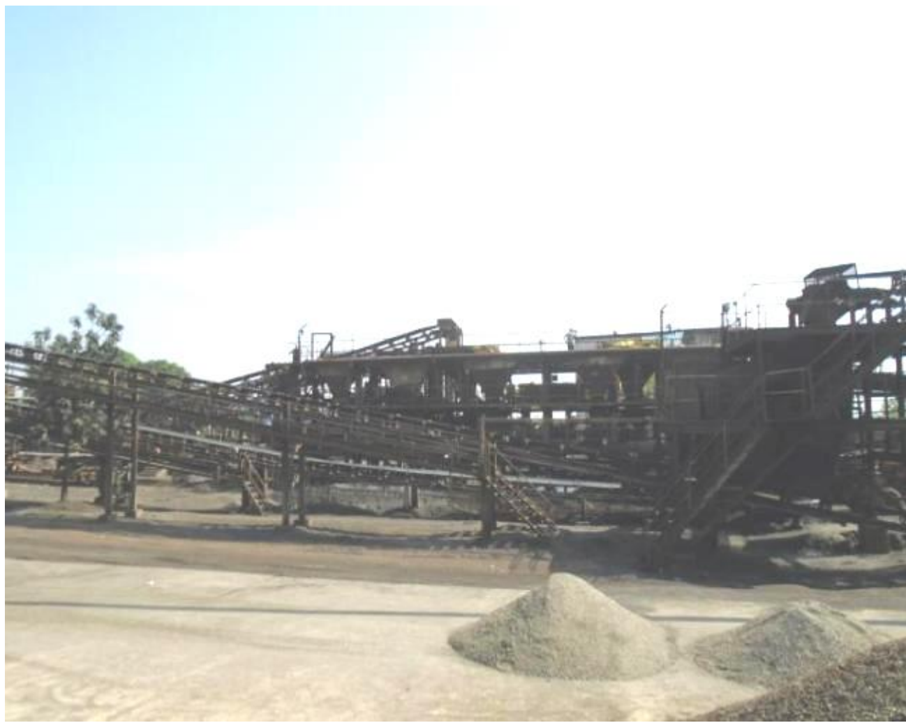
(figure 11: Jigging Plant)
