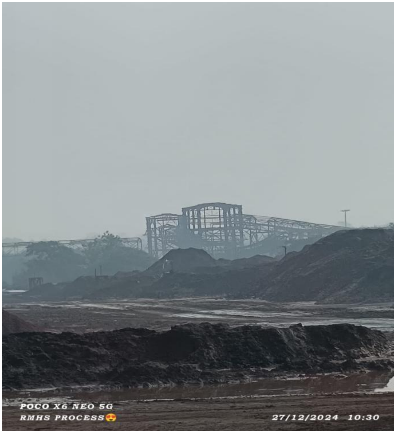
(Figure 6: Water Sprinkler - Iron Ore Yard)
