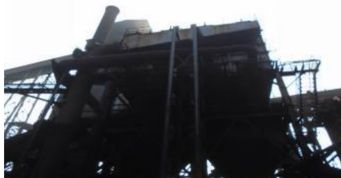
(fig. 8: DRI New Bagfilters - Cap:85,000m 3 /hr)
